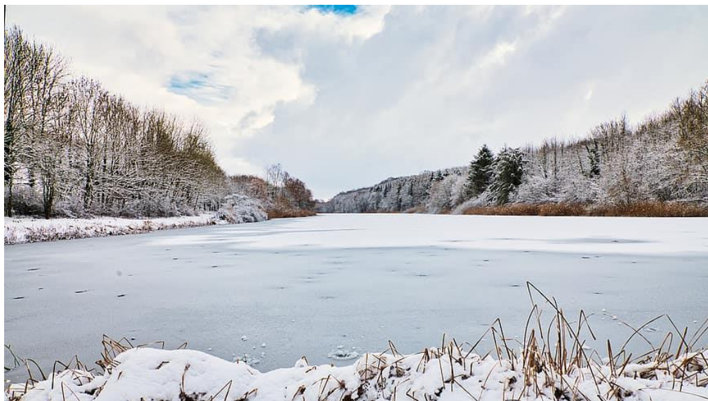
Figur 5-3 Fordrøyningsdam under vinterforhold (80)
