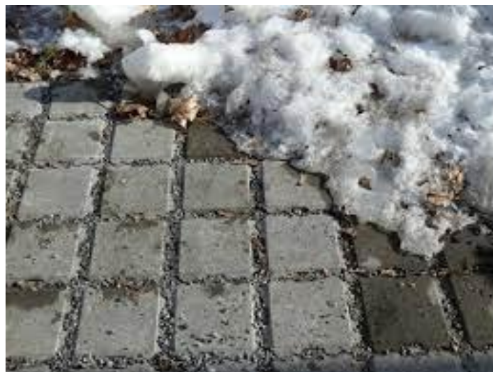
Figur 5-5 Permeable flater under vinterforhold (82)
