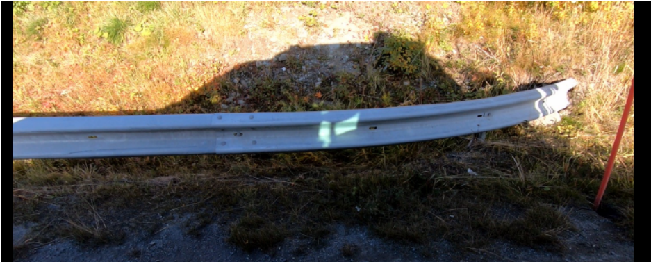
Figure 6.3: Missing foot
