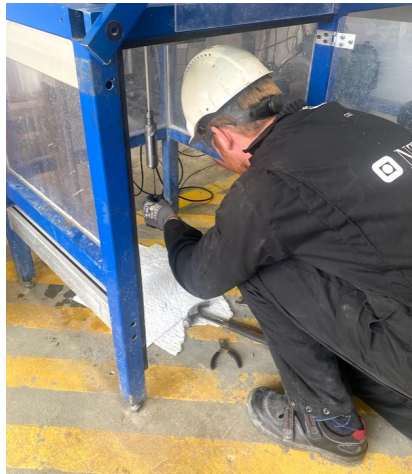
Figure 3.3: Team member with correct PPE under construction of the rig.
