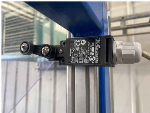
Figure 6.8: Stop button on hoisting system.
