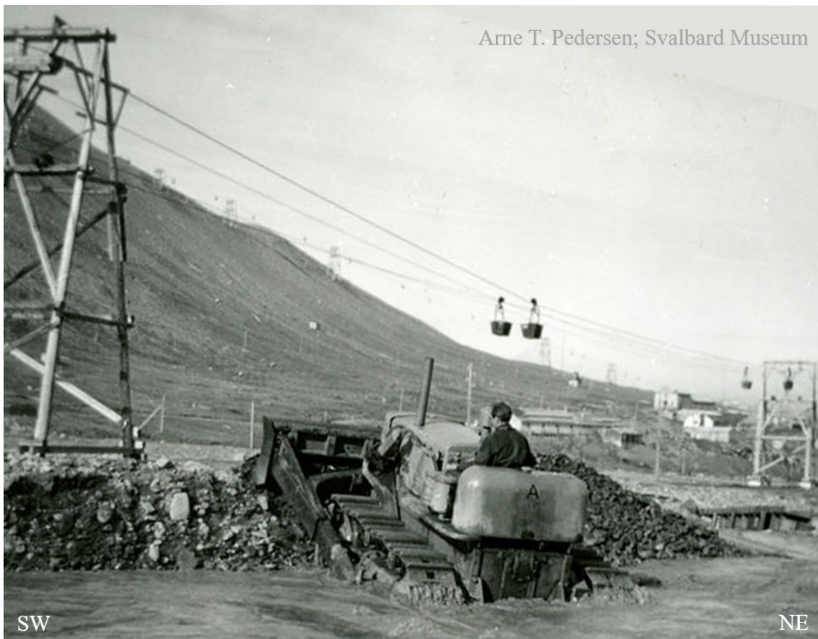
Figure 8: Crucial use of bulldozers to protect infrastructure along Longyearelva river dates to the 1950's (Pedersen and Svalbard Museum 1960). In this case is a bulldozer is used to keep the river from eroding the fundamentals of the cableway ramps used for transporting coal from the mines to the harbour.
