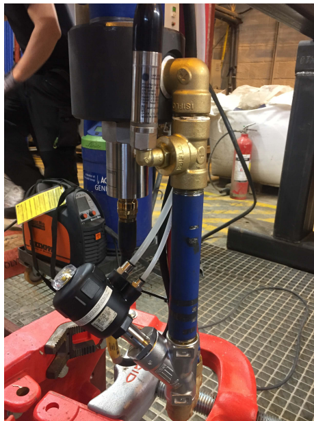
Figure B.3: Casing bottom with magnetostrictive, temperature and pressure sensors. Flow loop valve with control tubes
