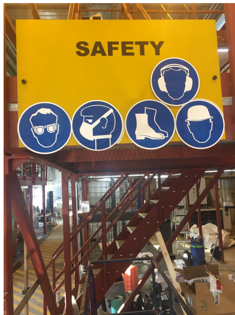
Figure B.1: Safety board instructing required personal protective equipment (PPE) during construction of the experimental infrastructure. From left: Eye protection, Breathing mask, protective footwear, hard hat and hearing protection above.
