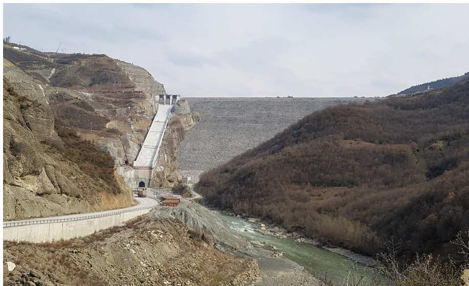
Figure 4.1. Moglice dam and spillway (Photo: Runa B. Frengen 27.03.2019)
