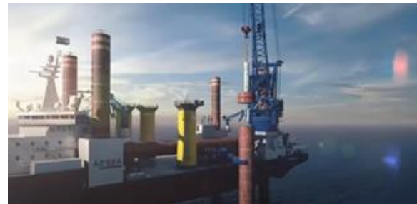
(b) Installation of foundations
