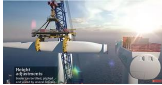
(f) Blade installation
