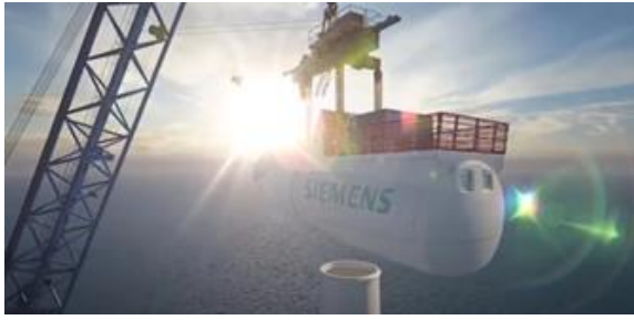
(e) Nacelle installation
