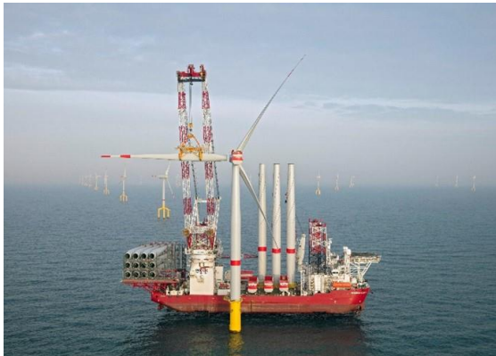
(a) Jack-up vessel installing a blade [25]
