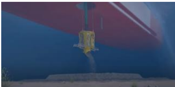
(a) Scour protection installation
