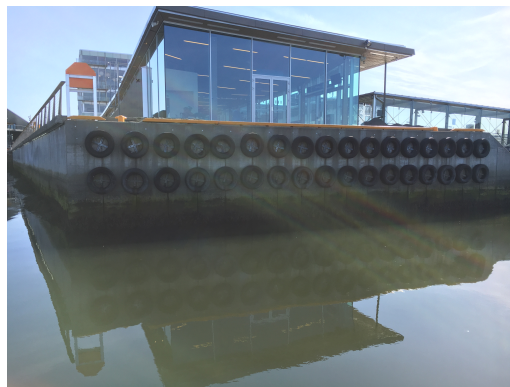
Figure 7.8: The tip of Hurtigbåttterminalen at which the berthing scheme was experimentally tested, depicted by the author. The width of the quay structure is approximately 18 meters.
