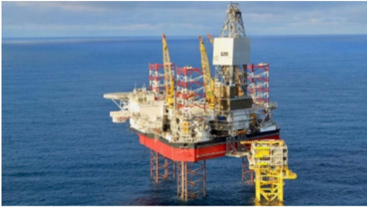
Figure 3.9: The unmanned Oseberg H Vestflanken 2 wellhead platform and the Askepott drilling rig [51].
