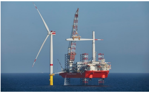
(a) Fred. Olsen Windcarrier's "Brave Tern" installing a wind turbine at the Albatros wind farm in the German North Sea (Renews Ltd, 2019)
