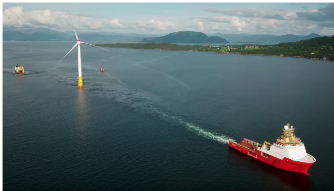
Figure 3.26: Towing of a turbine for Hywind Scotland (National Geographic, 2017)
