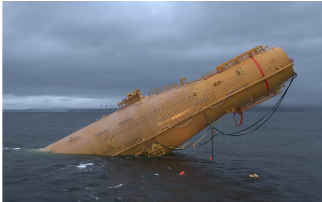
Figure 3.24: Upending operation of sub-structure for Hywind Scotland (Equinor, 2017)
