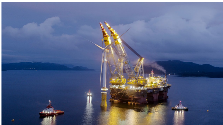
Figure 3.25: Heavy lift during mating operation by Saipem7000 (Equinor, 2020)
