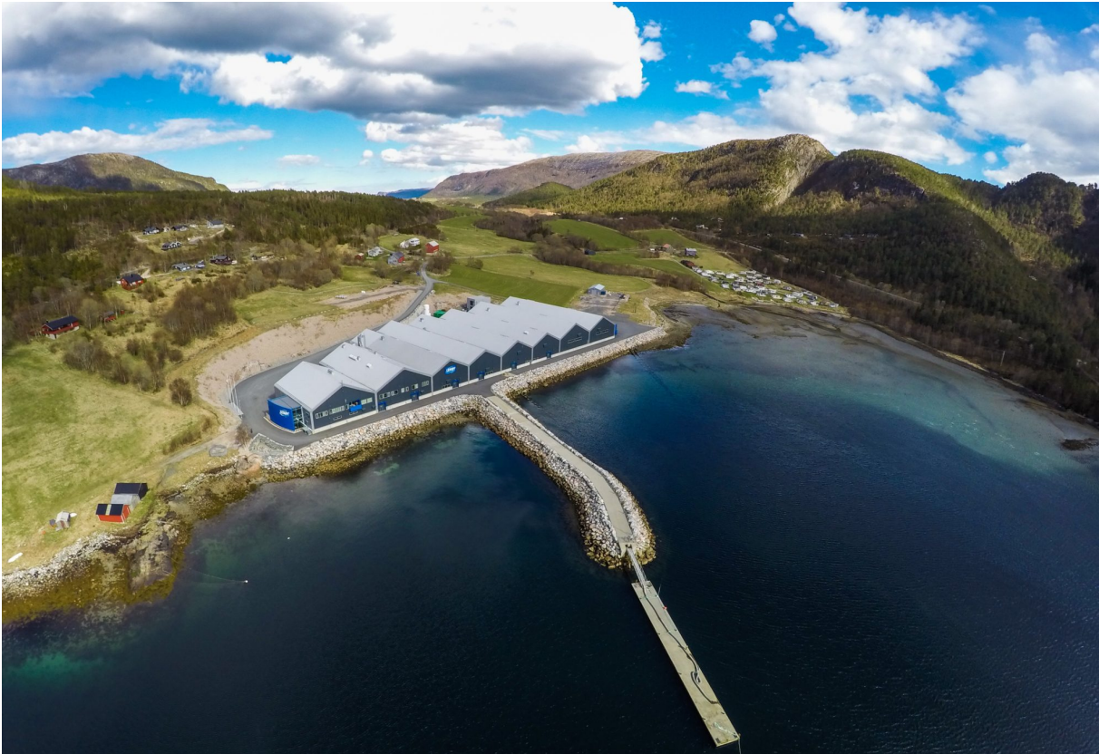
Figure 4.1.2: Lerøy's RAS-controlled hatchery in Belsvika, which for a brief time was the world's largest land-based aquaculture facility (Gemini (2017)).
