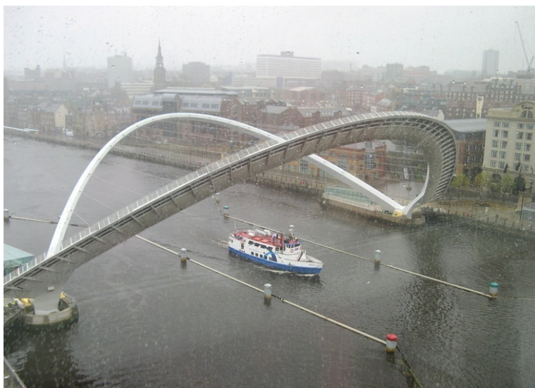
Figur 3.10: Gateshead Millennium Bridge (Davies, 2009)
