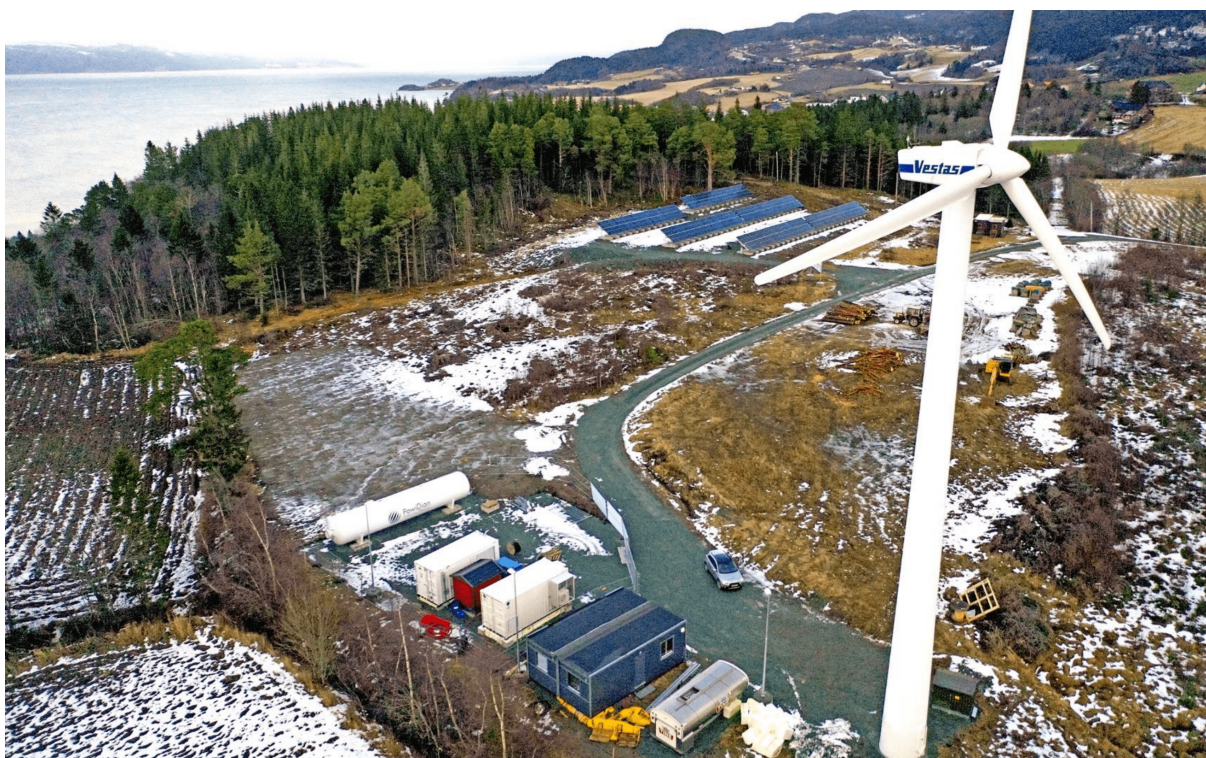
Figure 6.5: The technical installations in the microgrid at Rye [100].
