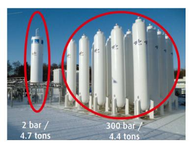
Figure 2.12: Illustration of Liquid and compressed hydrogen storage tanks [77].
