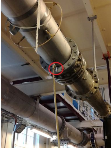
1i - Inlet pipe draining valve
