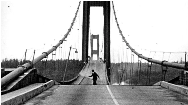
Figure 2.1: Tacoma bridge collapse, November 7, 1940. ( https://kiro7.com/ )
