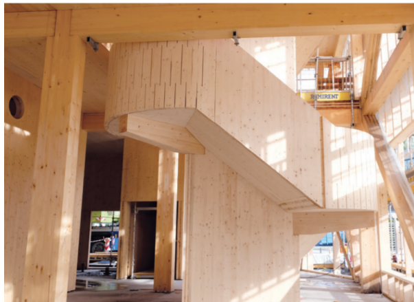
Figure 3.3: Picture of the staircase from the building site [28].
