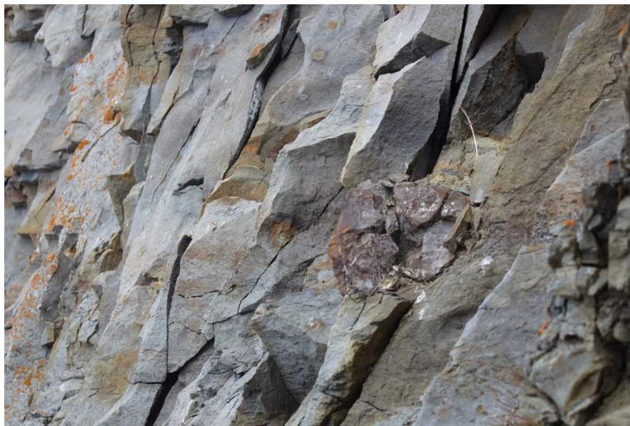
Figure 39 Closeup of the rock outcrops without any water sign
