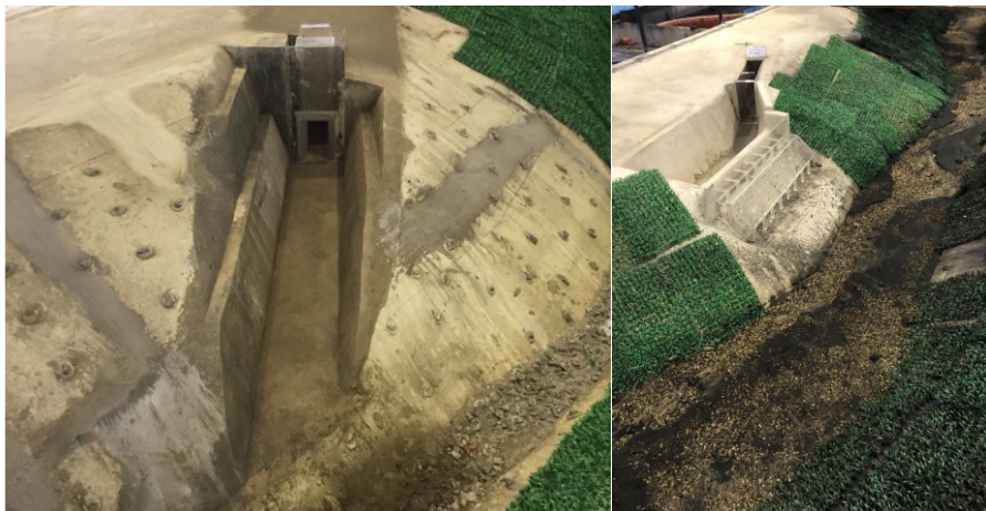
Figure 4.10 Initial SBT (left) from report ANNEX H-3 and modified SBT intake (right) (Adapted from report ANNEX H-2)
