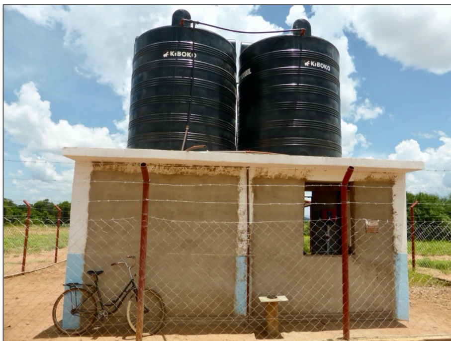
Figure 11: Water tanks at Isene pumping station
