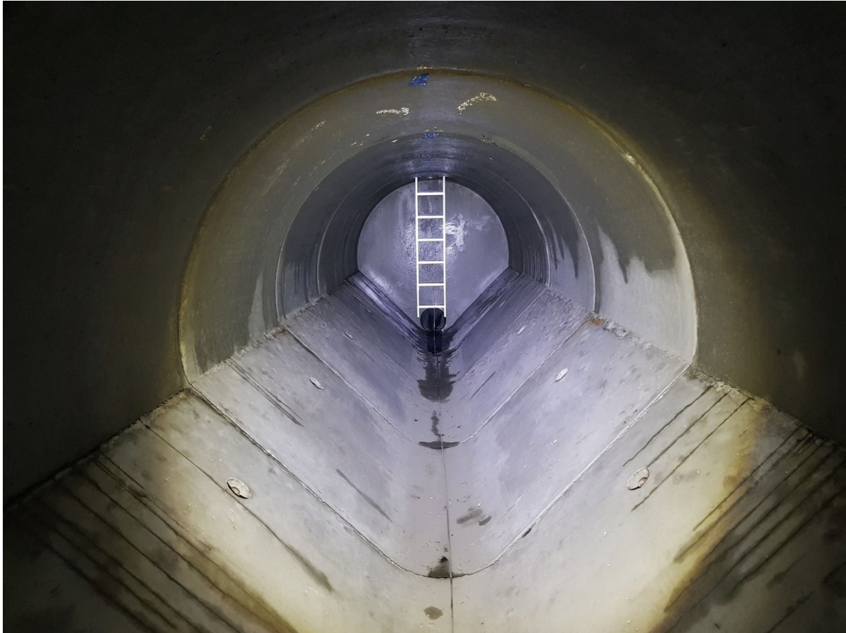
Figure 4.9: Inside of the detention basin looking north.
