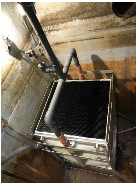
Figure 3.8 One of the membrane modules in the pilot plant. Courtesy of Tobias Hey.
