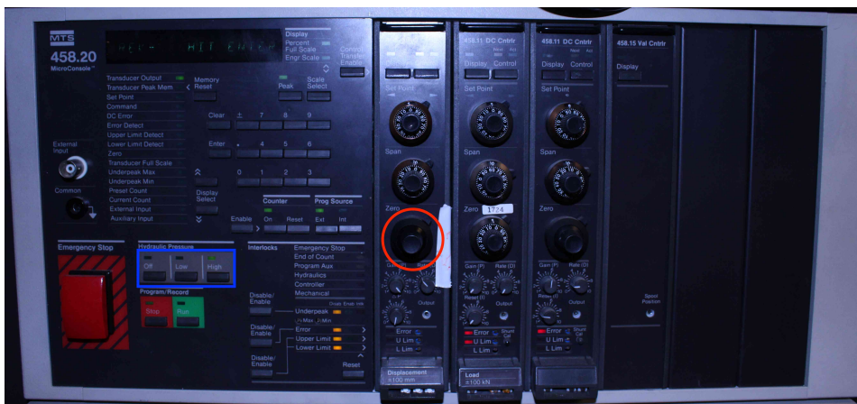
Figure 4.9: Load cell panel.
