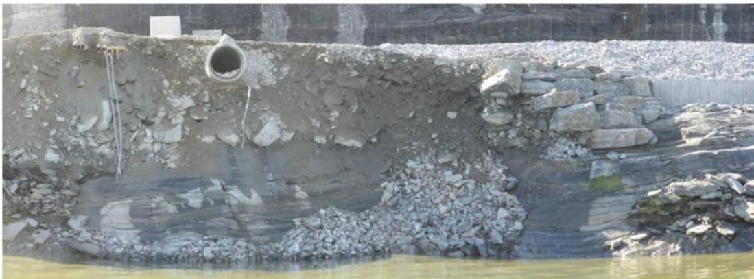
Figure 28: A photo from the seaside shortly after the landslide. Shows the northern part of the area where the pier reached land and the cuttings that passed through the road and the landfill. (Photo: Norut, ISBN 978-82-7492-305-8 report).
