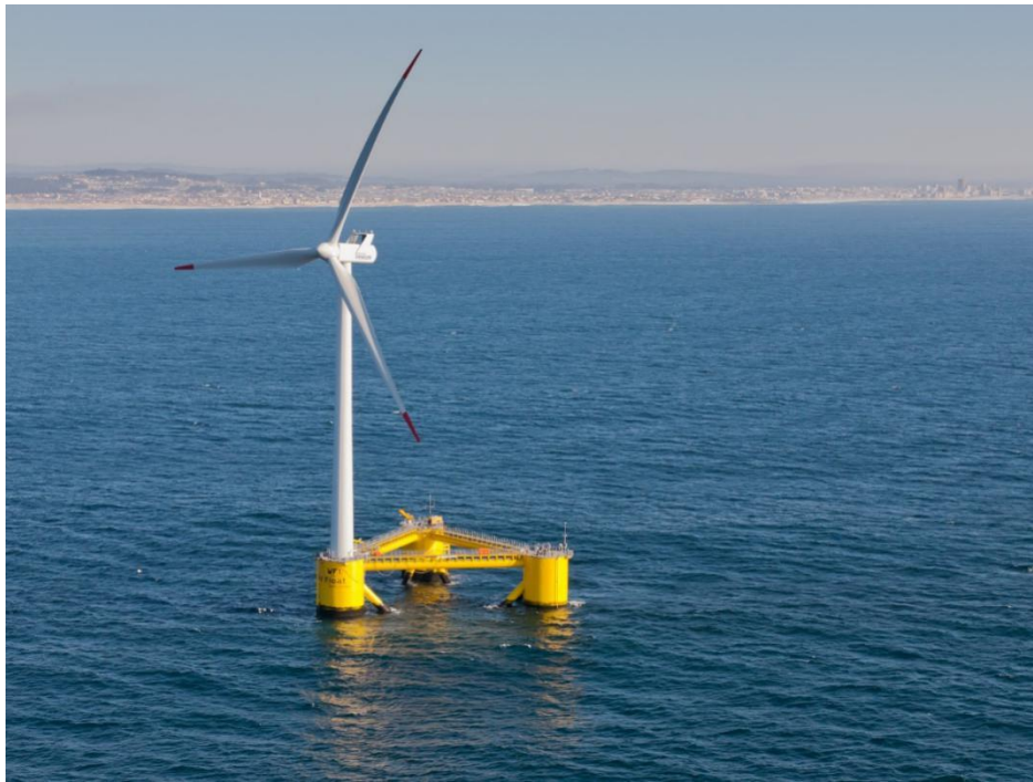
Figure. 1. An example of FOWT in offshore operation.
