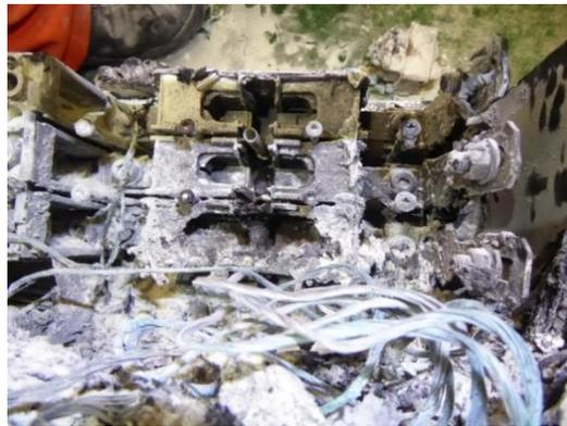
**Figure 1-1: Arc flash in a contactor, courtesy of BW Offshore.**
