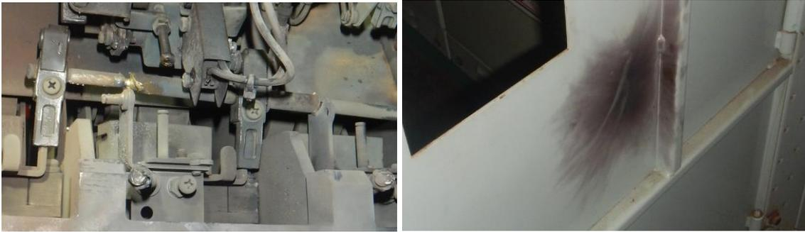
**Figure 1-2: Arc flash in air circuit breaker contacts, pictures courtesy of BW Offshore**
