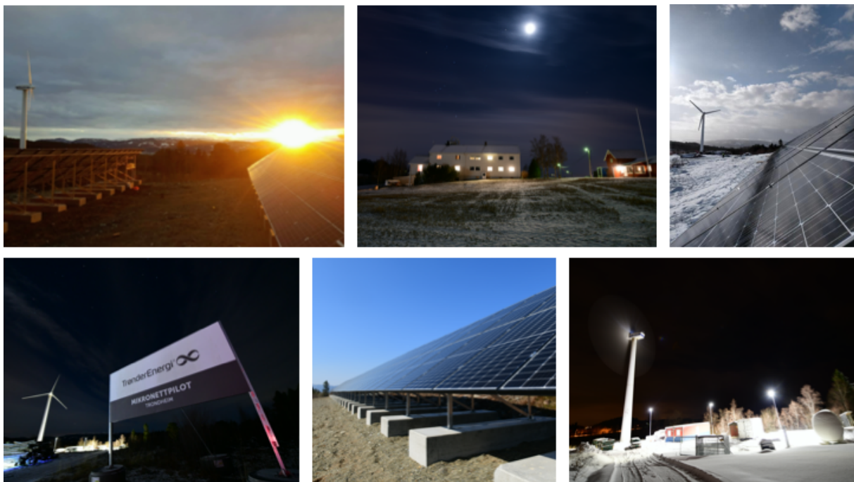
Figure 3.1: Pictures of the microgrid being set up at Rye, Norway. Taken by Bernhard Kvaal, TrønderEnergi.
