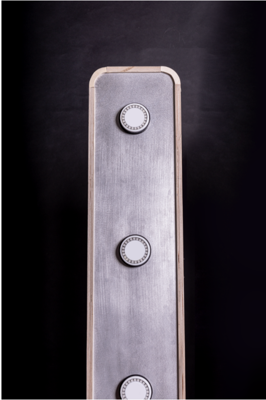
Figure 1: Close up look of one of the columns
