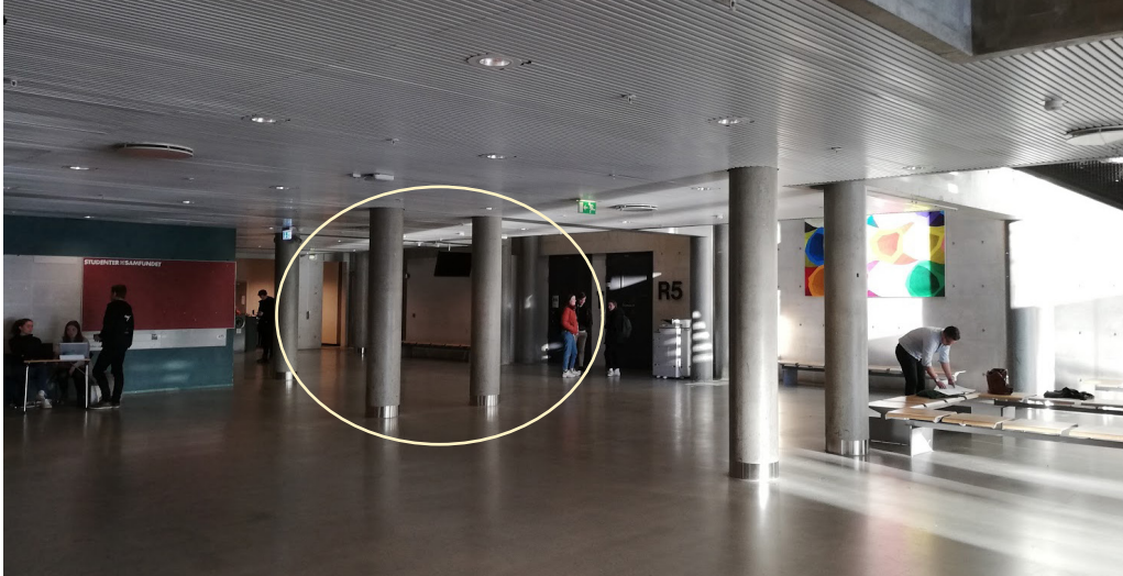
Figure 5.6. Open meeting area at NTNU Gløshaugen. The columns in question are circled.
