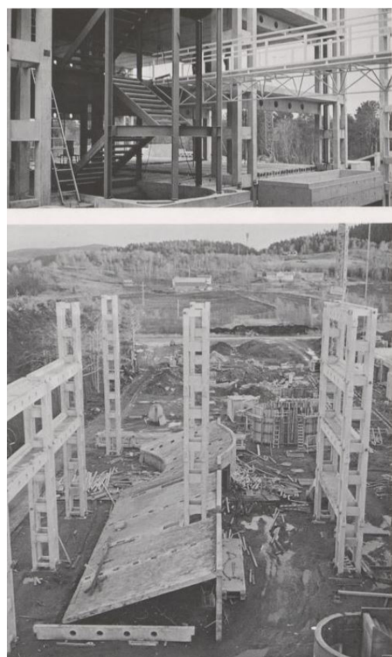
Figure 16. Concrete structure shown during construction
