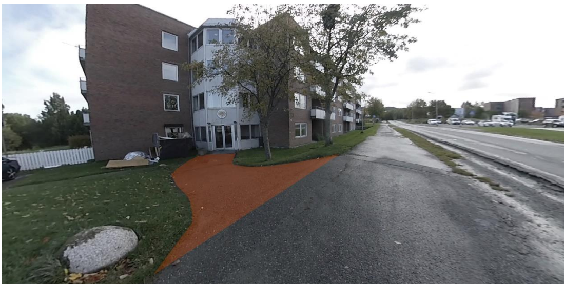
Figure 18. Slope area with slipping risk during winter
