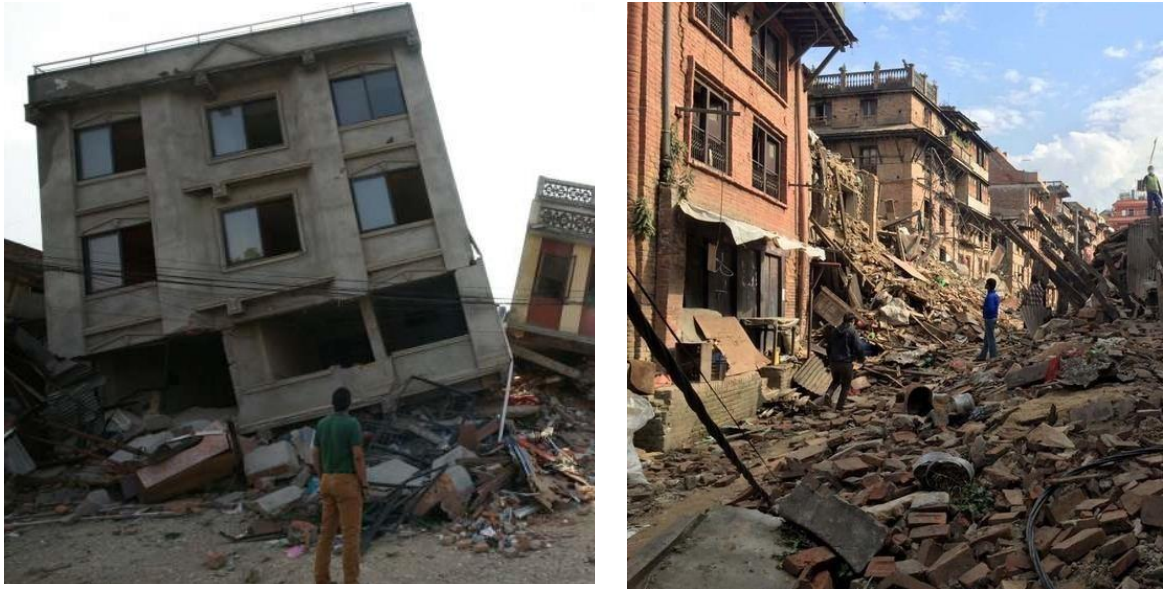
Figure 4:Kathmandu valley after Earthquake 2015
