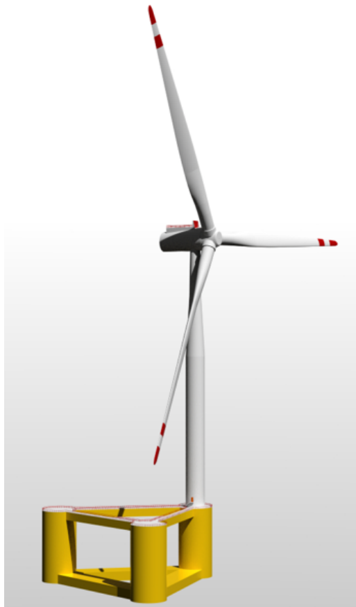
Figure 3.1: The WINDMOOR 12 MW FWT concept. Figure provided by Inocean.
