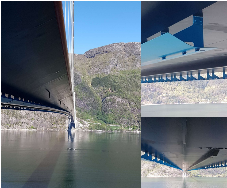
Figure 6: Aerodynamic details and vertical curvature of the Hardanger Bridge girder
