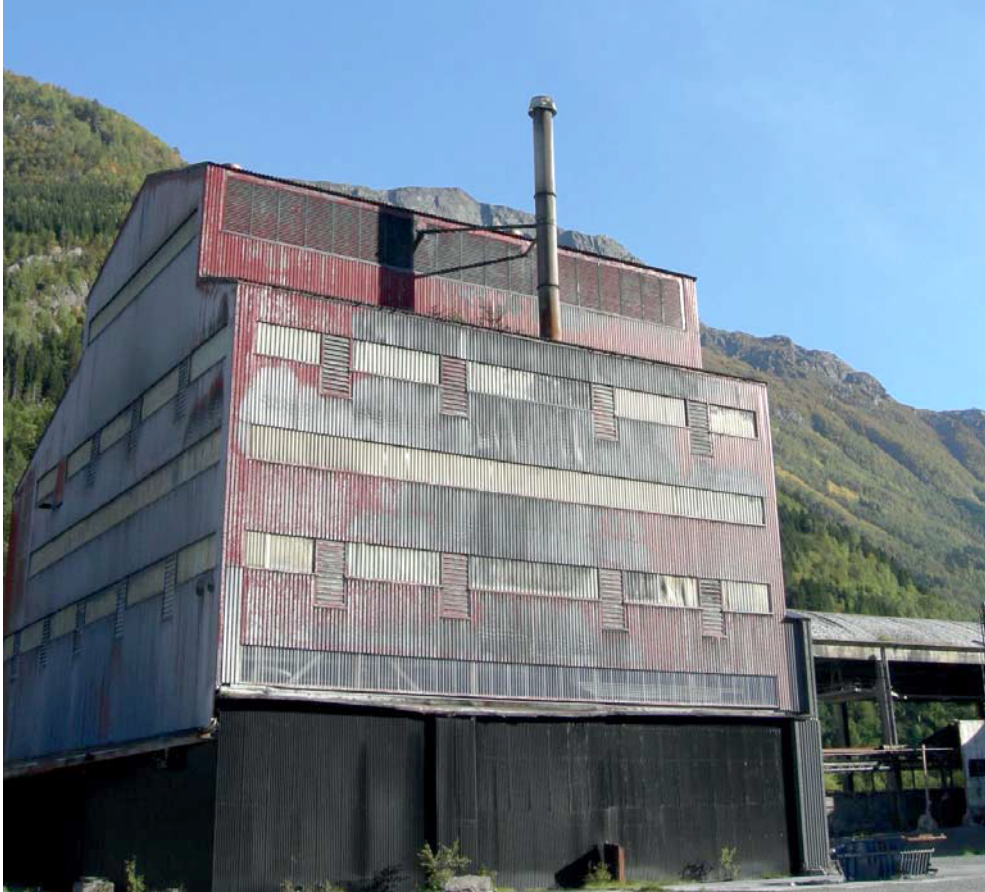
Figure 4.3 - Exterior shot of the house of furnace III. Built in 1976 and in operation from 1982, the furnace was listed in 2011 on the basis of technological importance. The red metal sheets store a furnace which was once the largest of its kind in the world.
