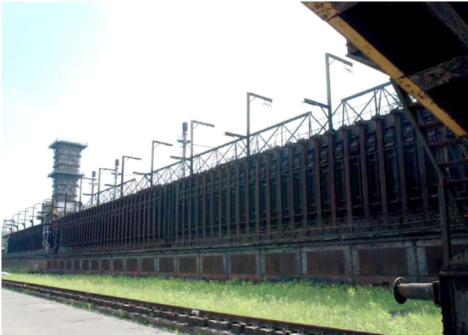
Figure 3.2 - 'Black side' with rows of coke ovens. Quenching tower where coke was cooled with water in the background.
