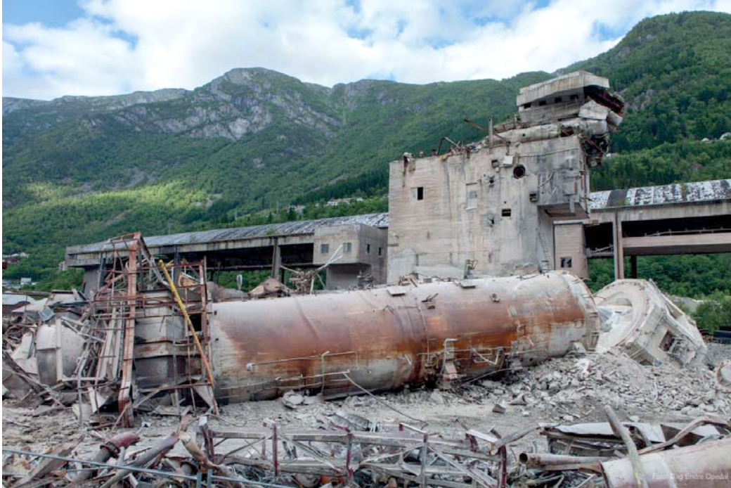
Figure 4.5 - The tallest of the two lime kilns was knocked down on the 25th of July 2012. The lime kilns lacked the international significance and were considered expendable in so far as the demolition of the kilns would not jeopardize the World Heritage bid. Photo: NVIM/Harald Hognerud.
