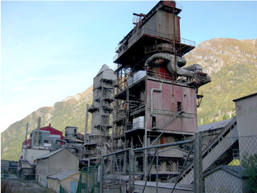
Figure 4.1 - The southern end of the smelter site as of September 2010. Lime kilns in the front and the red carbide furnace in the far back. Today the fences have been removed along with most of the buildings.
