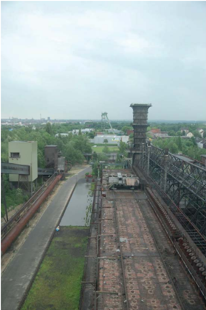
Figure 3.4 –The detached gaze. Kokerei Hansa from above. Navigable conveyor bridge to the left.
