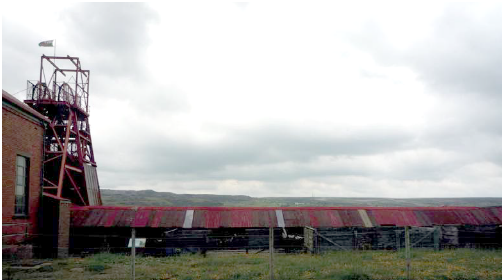
Figure 5.1 - Big Pit National Coal Museum with the steel headgear to the left
