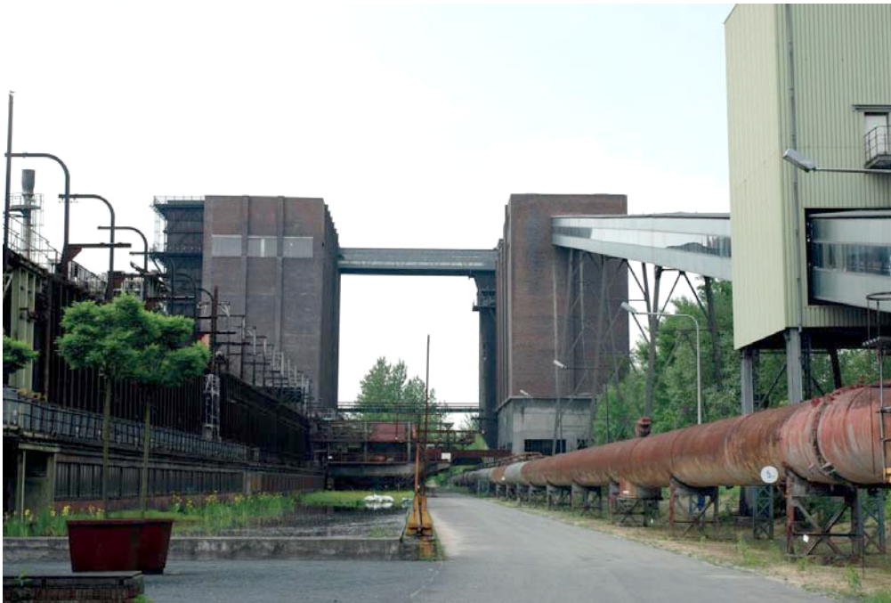
Figure 3.3 - Kokerei Hansa with navigable conveyor bridge to the right. Coal tower (left) and coal sorting tower (right) in the back.
