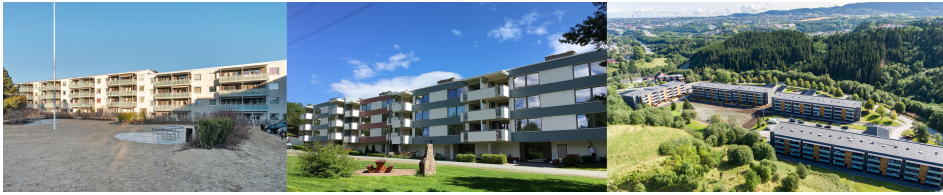
FIGURE 5.2. Examples of a typical apartment block.
