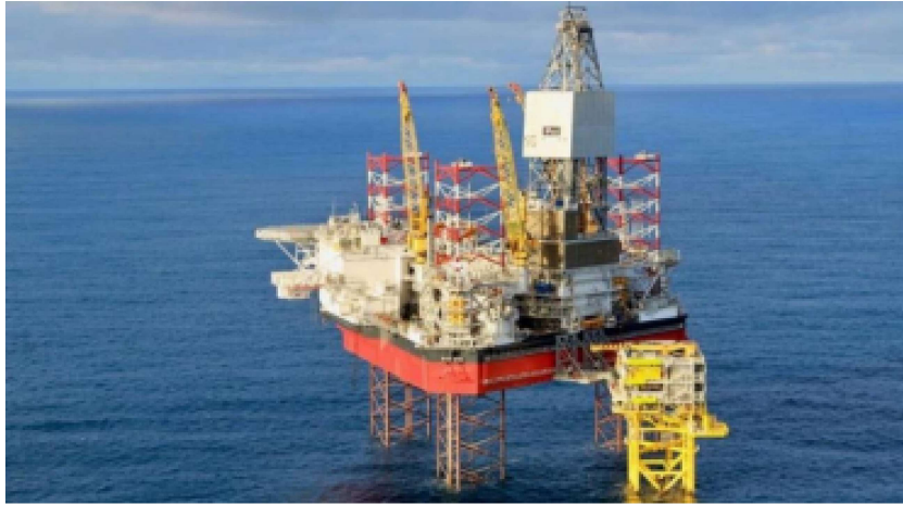
Figure 3.9: The unmanned Oseberg H Vestflanken 2 wellhead platform and the Askepott drilling rig [51].
