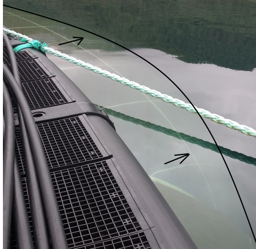
Figure 4.8: Black line marks the visible edge of the skirt being lifted due to the current. Black arrows indicate the main current direction. Overlap is visible just beneath the bottom arrow.
