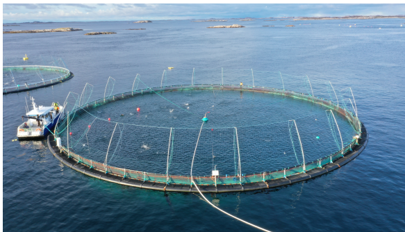
Figure 1.3: Cage at SINTEF ACE facilities Rataren, Frøya, Norway, with a diameter of 50 m showing the floating collar, feeding system and the cage net strung up on the inside (green net). (Photo: Magnus Oshaug Pedersen, SINTEF Ocean, shared with permission).
