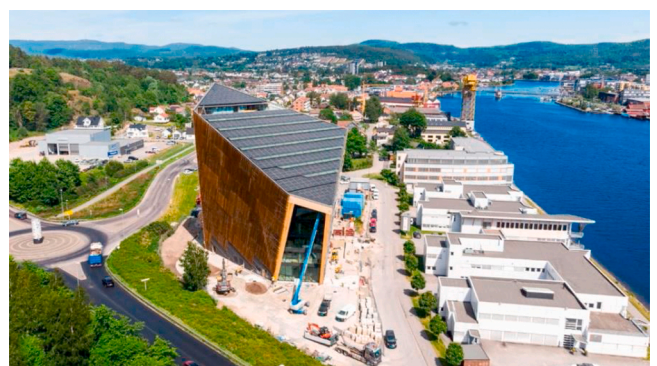
Fig. 5. Powerhouse Telemark exterior during construction. Image courtesy of Skanska.
