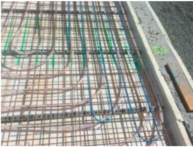
Fig. 6. LowEx hydronic pipes before poured concrete slab. Image courtesy of Skanska.
