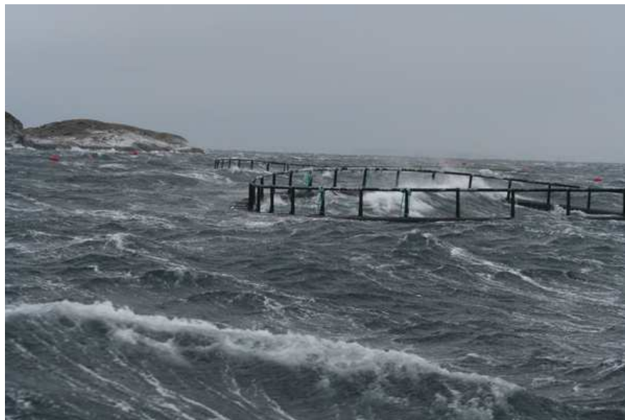
Figure 1.2: Open cage fish farm of the circular collar type in Flatanger, Norway. The photo is taken during the winter storm Narve in January 2006. Large elastic deformations of the structure are seen. (Photo: Marius Dahle Olsen)
