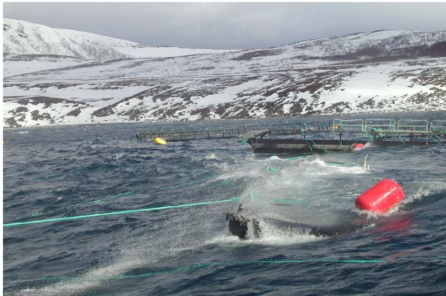
Figure 1.8: Example of a collapsed fish farm after a storm, with large fish escape as a result.
