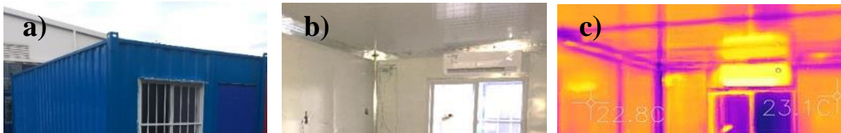
Figure 3. a) Standard container building, b) Test of Vacuum Insulation Panels (VIP) with thermocouples and heat flow meters, c) Thermogram of the walls before the installation of VIP.
