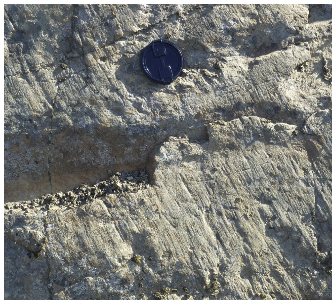
Fig. 7. Clearly visible striation in sliding direction on the lower section of the exposed sliding surface of Revdalsfjellet 1. Foto: H. Bunkholt (NGU).
