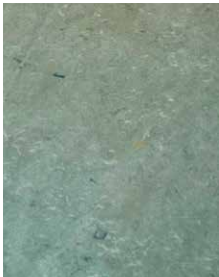
Skvett puss, malt tapet, malt betong, linoleum
