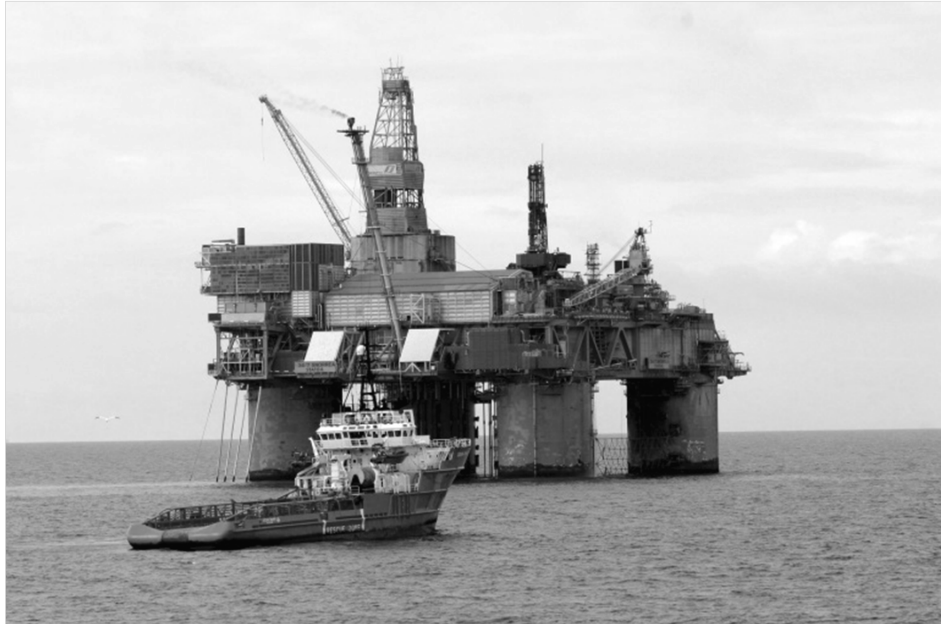
The Snorre Alpha Platform is still in service today, almost ten years after the blowout (Photo: Rune Johansen/Statoil)
