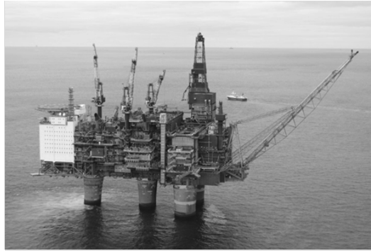
Statoil's Gullfaks C platform in the northern part of the Norwegian North Sea. (Photo: Øyvind Hagen/Statoil)
