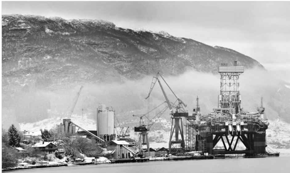
Two fatal accidents occurred on the semi-submersible drilling rig Scarabeo 8 at Westcon Yard in Ølensvåg in 2009 and 2011. Both were investigated by the NLIA (Photo: Håvard Sæbø)
