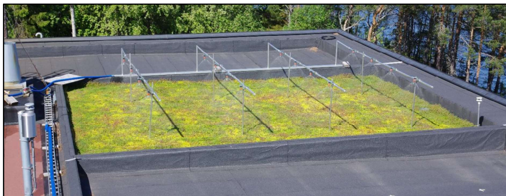
Figure 4 Rainfall simulator over the detention-based green roof on 11.6.2019.
