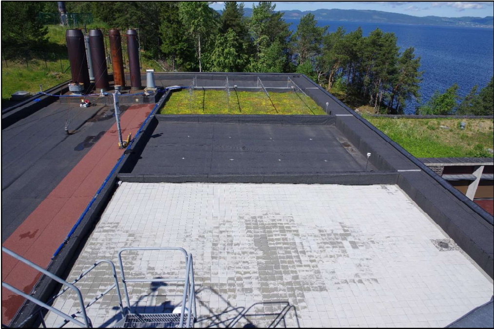
Figure 3 Three different rooftops at Høvringen on 11.6.2019. NB.: each of the rooftops with size 8 \times 11 meters receives additional stormwater from surrounding separation walls and parapets with an area of 12\text{m}^2 .
