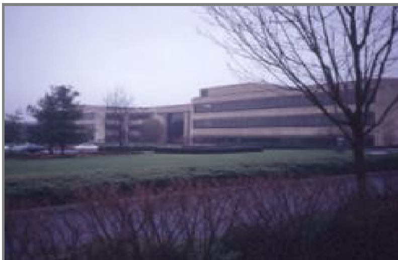
Bilde 11: Foster Wheeler. Perryville, New Jersey, USA.
