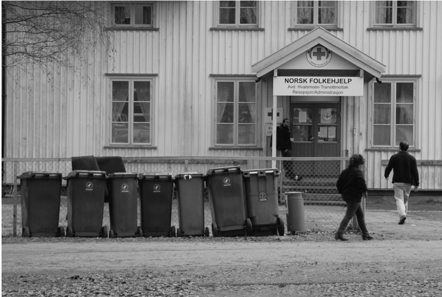
Figure 8.2 Entrance. Photo: Karine Denizou.
