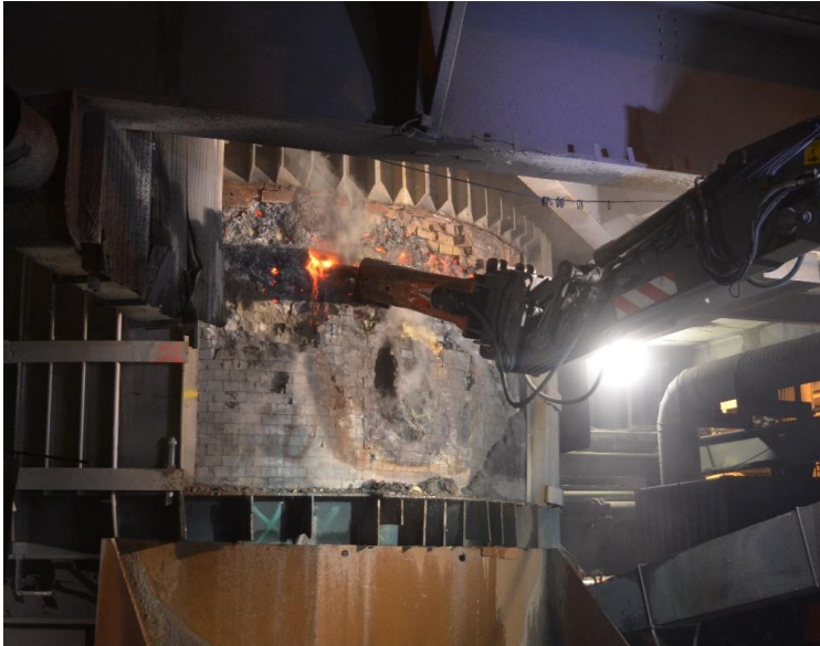
Figure 161: Photo taken during excavation of a 75% FeSi furnace at Finnjord.
