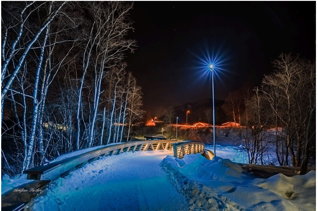
Figure 16: Evjen Bridge. Photo: Arnfinn Sæthre
