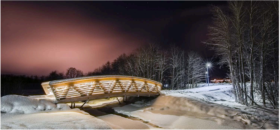
Figure 17: Follo Bridge. Photo: Arnfinn Sæthre
