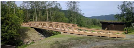
Figure 13: Evjen bridge-. Structural bridge in the center, Curved platform on both sides.
