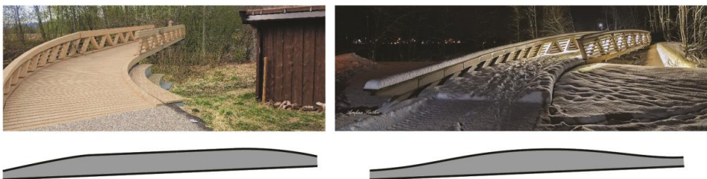
Figure 49: Rather late in the design process, the top chord shape was changed due to structural requirements.
