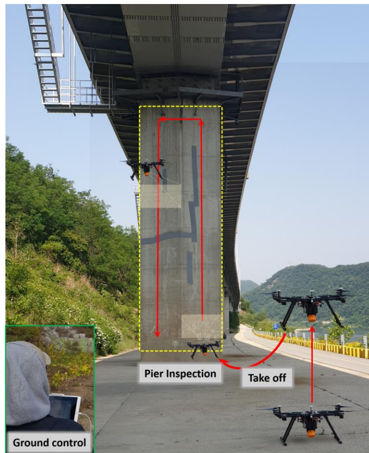
Figure 13. Experimental setup and inspection procedure of bridge pier
